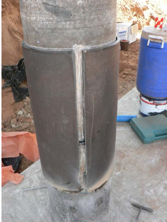
Photo 7 – Steel sleeves around piles to be jacked
