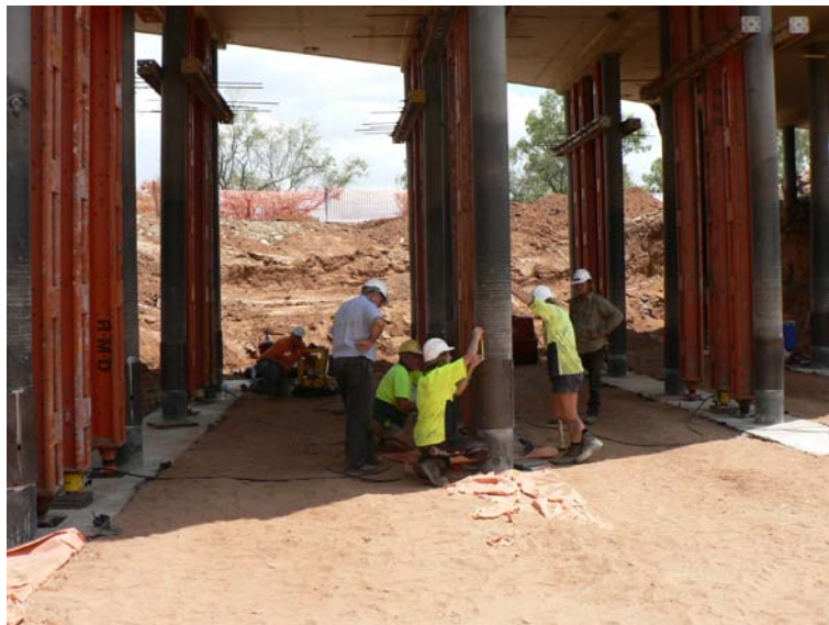
Photo 8 – Measuring the amount of displacement
