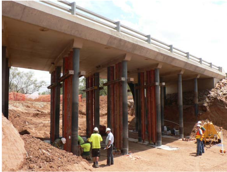
Photo 5 – Scorpion Creek Bridge Jacking
