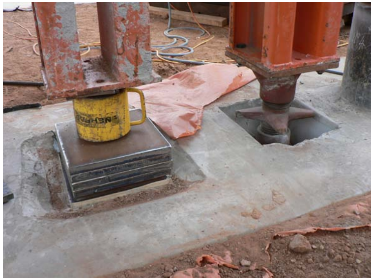
Photo 6 – Hydraulic jack and Maegashore support
